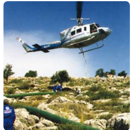
Fig. 27 Pipelaying by helicopter, PE-Xa Courtesy of Golan
