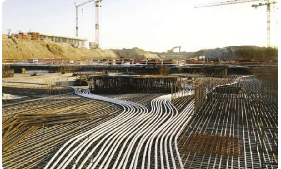
Fig 14. Geothermal heating system, PE-Xa
