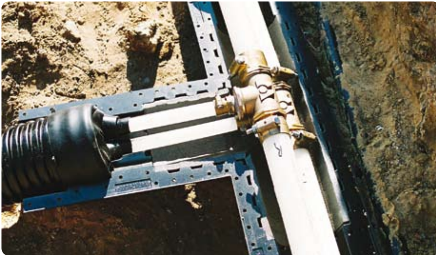
Fig 15. District heating system, PE-Xa
